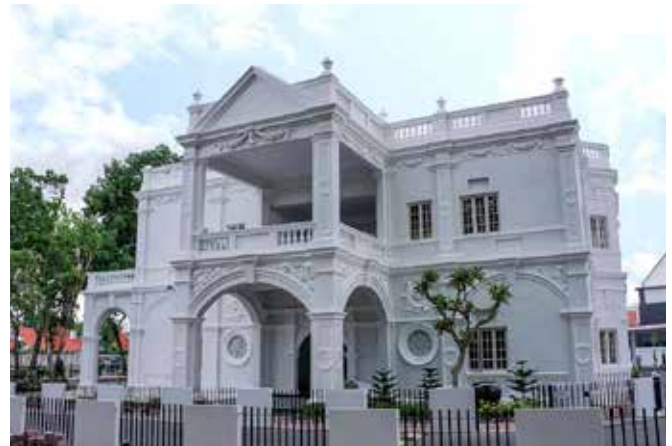
Restored ornate façade of the Karikal Mahal at 25 Still Road once again awes visitors and passers-by. Photo courtesy of The Straits Times
