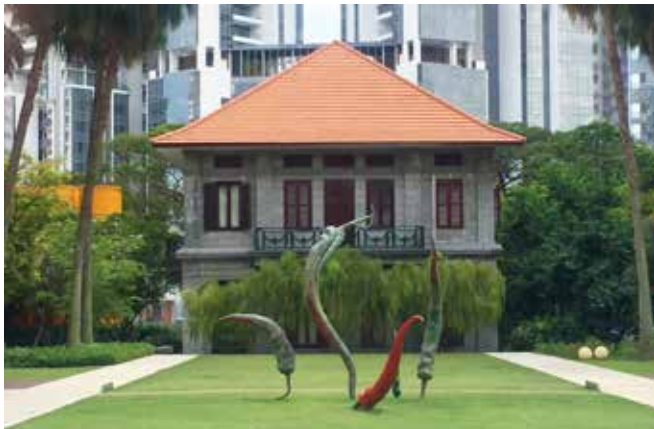
The Pavilion, restored to its former glory with support and guidance from the URA, has become a clubhouse overlooking the condominium's pool.
