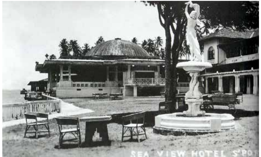
The majestic colonial bungalow of the old Sea View Hotel was Katong's landmark in the early 1900s. A condominium now stands on its site in Meyer Road. Photo courtesy of Joo Chiat, A Living Legacy by L Kong and TC Chang
