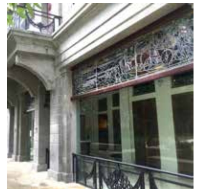
Carefully restored stained glass panels, depicting nautical and Middle-Eastern scenes, point to the Baghdadi Jewish origins of the Elias family. Ornate cast-iron balustrades at the verandas got new glass walls to comply with modern safety requirements.
